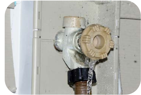
Leaks/Other Water Use
