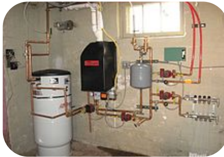
Hot Water Distribution Layout
